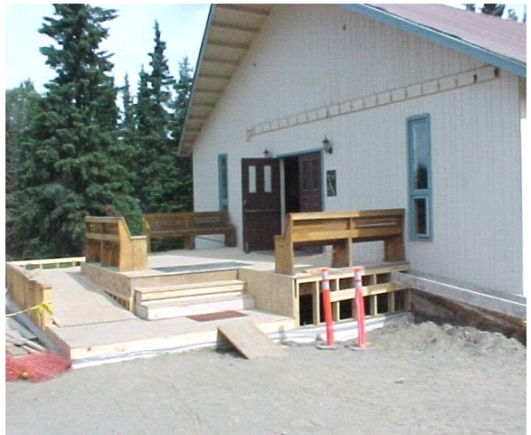
The new foyer area (without walls) and wheelchair ramp.
