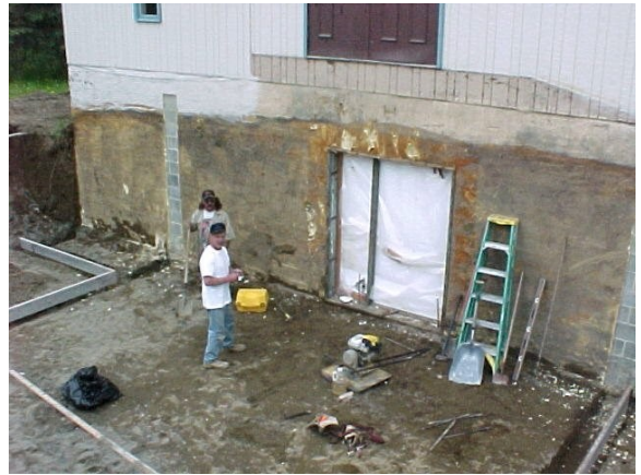
Gary Spruill and John Evanson preparing the slab area.
